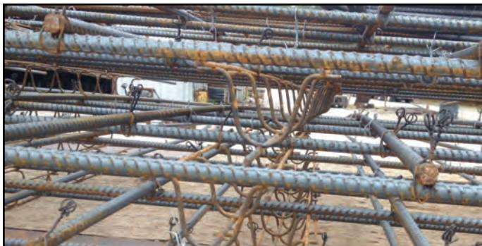
Another way we can make your job easier is for us to pre-tie the slab bolsters onto and in between mats for you so that they do not have to be shipped and installed on site.
